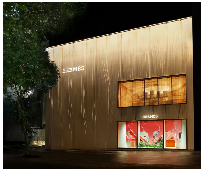
The renovated Lee Gardens store in Hong Kong reopened on 12 June 2024.
